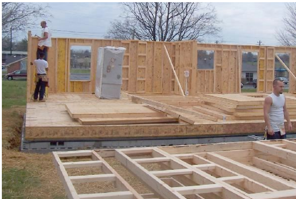
NHC pre-framed panels set up easily.
